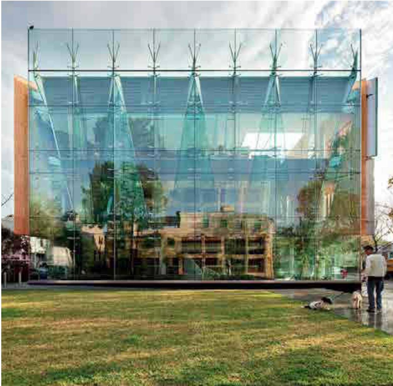
Glazed Facade with Planting for passive air renovation (Bio-Filter)
