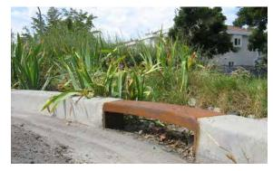
Example of sustainable design elements in the Carrall Street Greenway include storm water infiltration planter boxes, a permeable paver system, and rainwater channels
