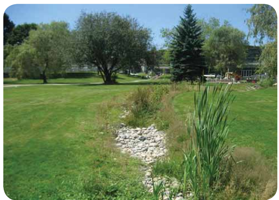
Stormwater Swale
