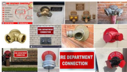
Examples of Fire Dept. Connections
