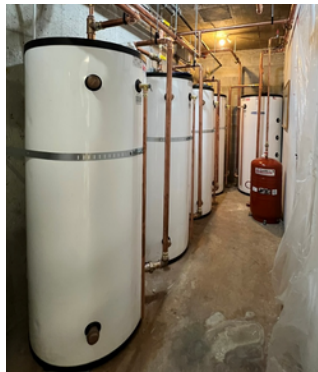
Hot Water Storage Tanks
