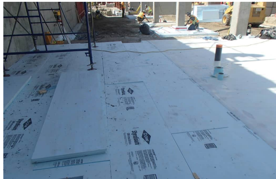
Figure 9: Below grade insulation
