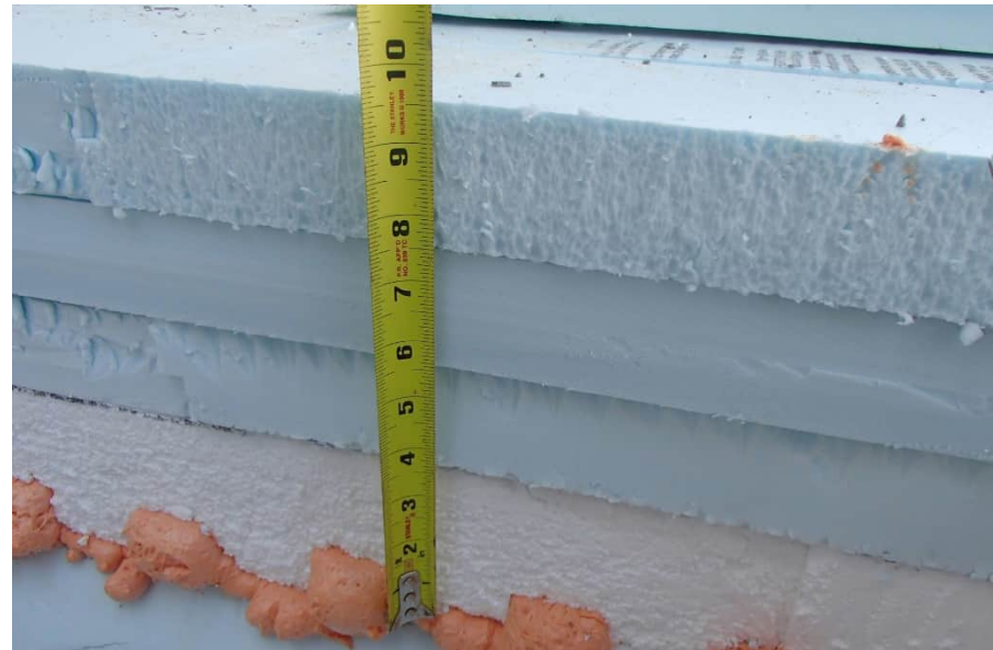
Figure 2: Photo demonstrating insulation thickness installed on site.
