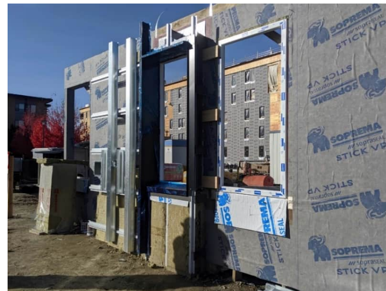
Figure 1: Mock-up wall illustrating window installation.
