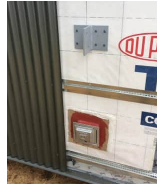
Figure 3: Mock up of typical air barrier penetrations.
