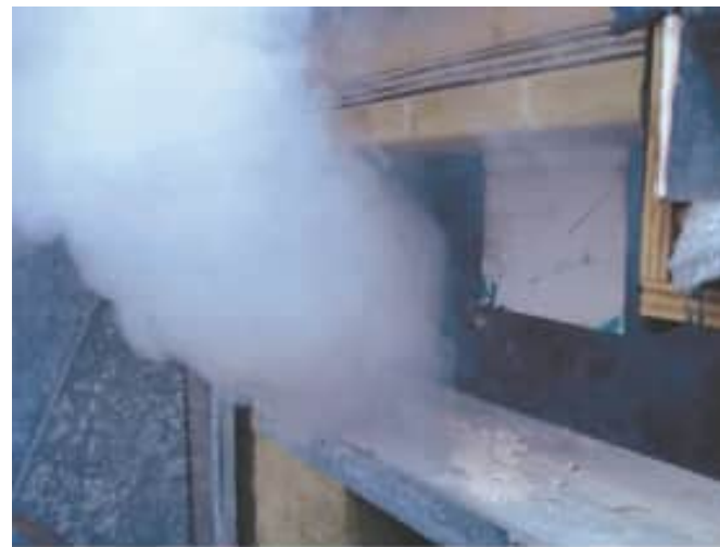
Figure 5: Qualitative smoke tracer testing of a parapet.
