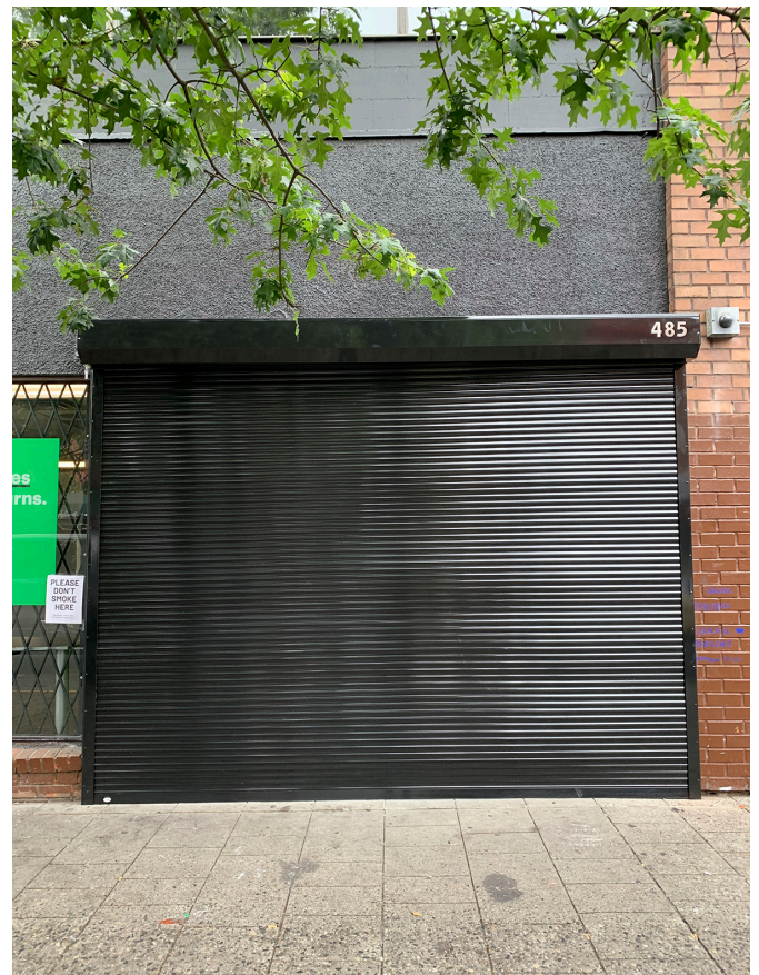
Exterior of THIS Gallery at 485 Main Street (now located at 268 Keefer Street) BEFORE rolling shutter gate installation.
