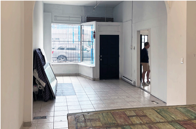
Interior of the site BEFORE renovations at 748 East Hastings.
