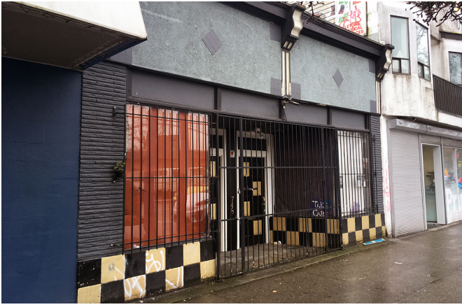
Exterior of the site BEFORE renovations at 748 East Hastings.
