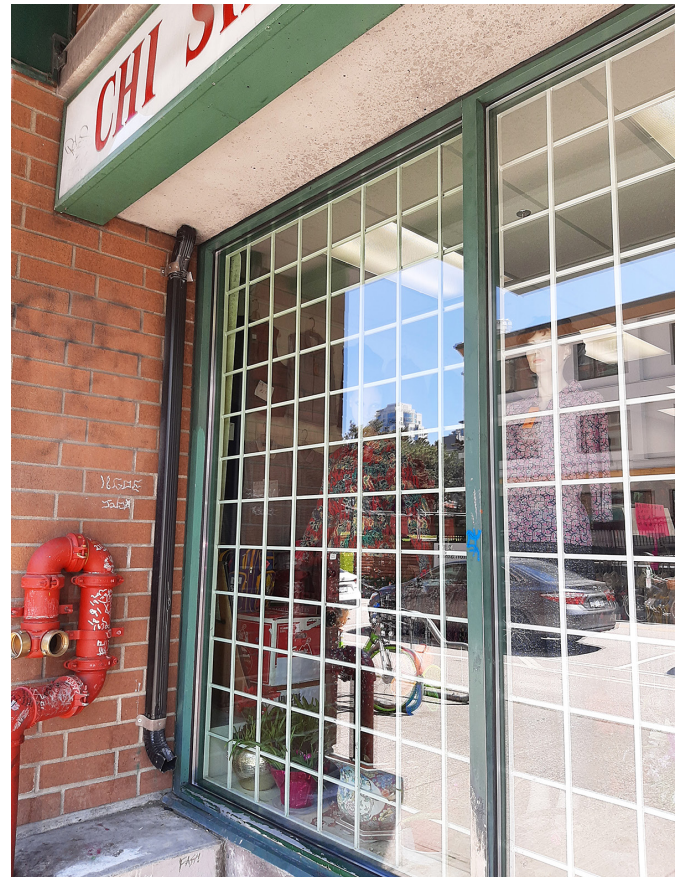
Exterior of Chi Shing Trading Co at 255 Union Street AFTER glass panel replacement.
