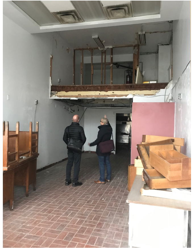
Interior of vacant space during renovations at 525 Gore Avenue.
