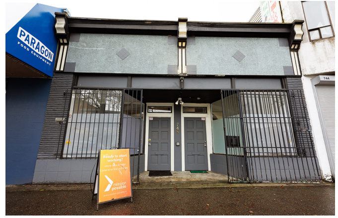
Exterior of the site AFTER renovations at 748 East Hastings.
