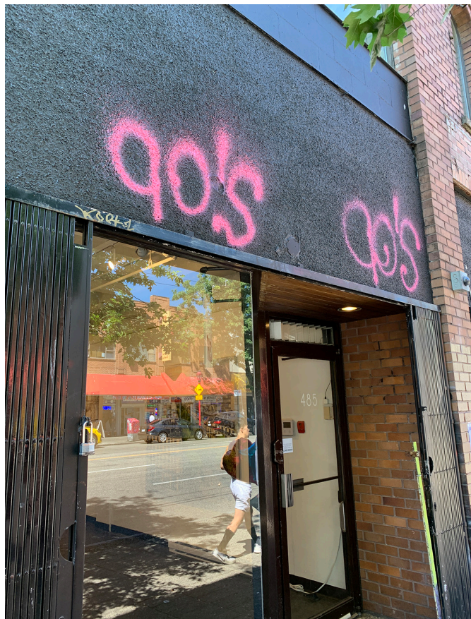
Exterior of THIS Gallery at 268 Keefer Street BEFORE rolling shutter gate installation.
