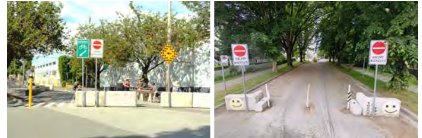
Figure 2 and 3: Examples of traffic calming measures with concrete barriers at Adanac-Vernon Plaza (left) and Yukon Street at W 12th Avenue (right)
