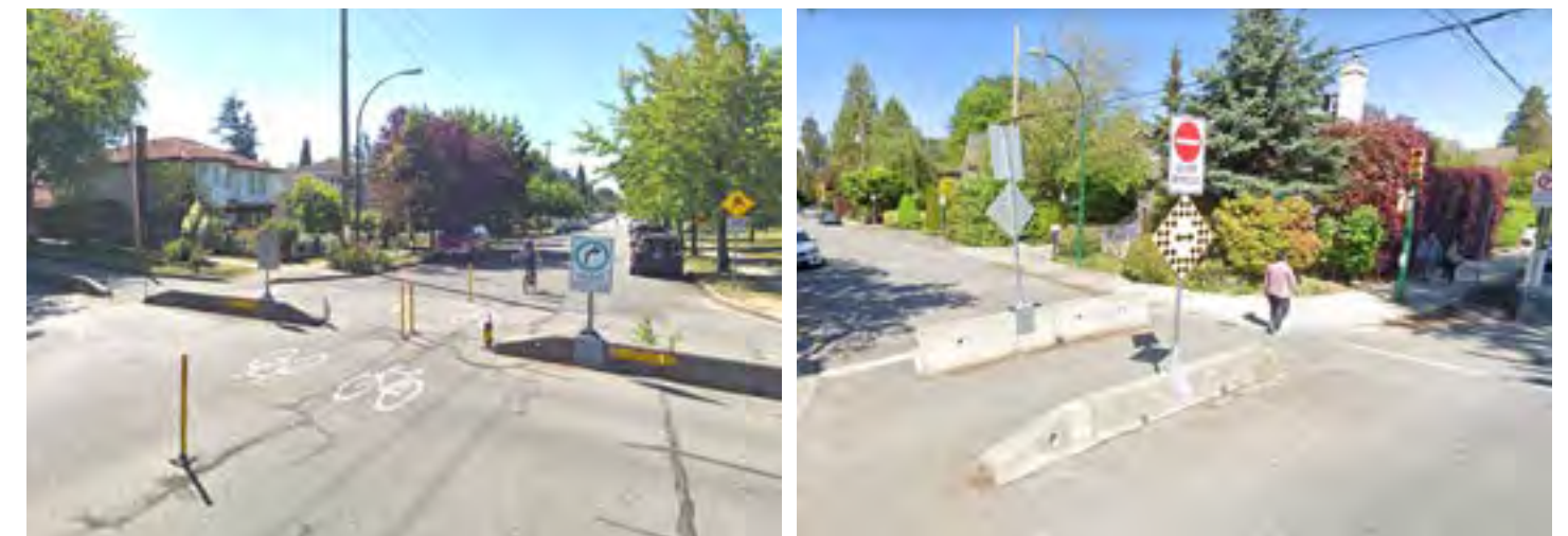
Figure 4 and 5: Examples of traffic calming measures with concrete barriers at Ontario Street at Peveril Avenue (left) and Macdonald Street at W 3rd Avenue (right).
