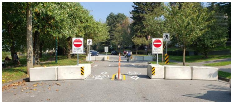
Figure 1: Photo of temporary traffic calming closure at Wall St at Oxford and Cambridge Parks
