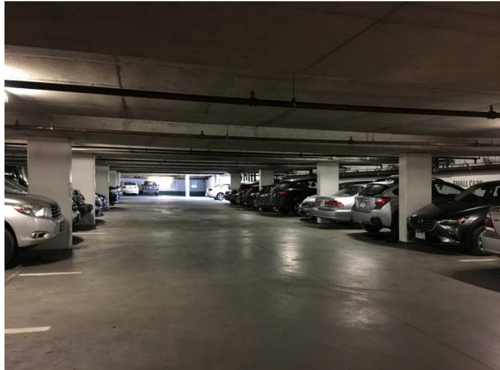
Under NFPA 13 the fire protection sprinklers for garages are typically designed to “Ordinary Hazard Group 1” which is defined as occupancies where combustibility is low, quantity of combustibles is moderate, stockpiles of combustibles do not exceed 8 feet (2.4 m) and fires with moderate rates of heat release are expected. Other examples of Ordinary Hazard Group 1 are restaurant service areas, automobile showrooms, and bakeries.
