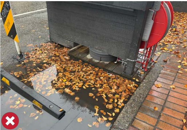
Photo 35: Curbside patios with inadequate drainage
