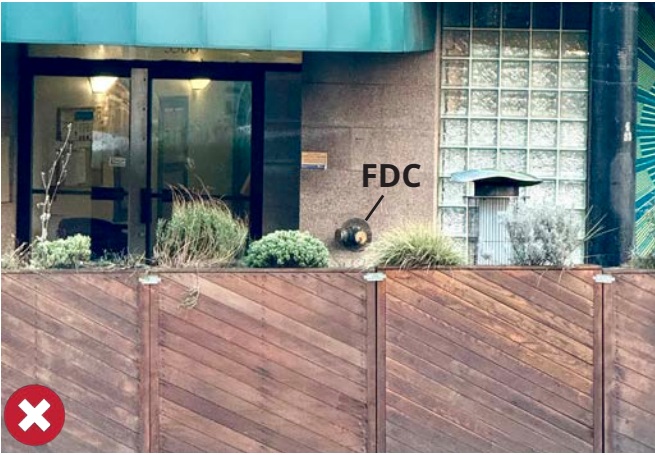
Photo 38: Does not meet minimum clearance of FDC
