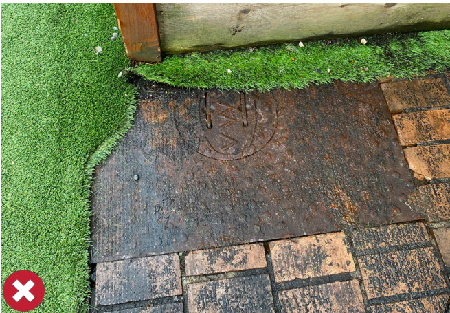
Photo 36: Patio covering in-ground utilities
