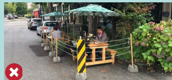
Photo 14: Railing lacking structural integrity
