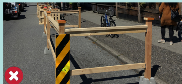
Photo 13: Railing with large opening
