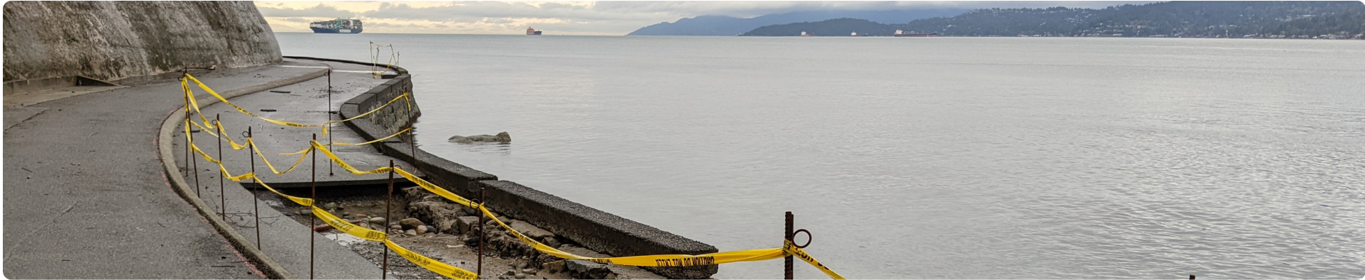
▲ Damage to the Stanley Park seawall following king tides and stormy weather (Source: Vancouver Park Board)
