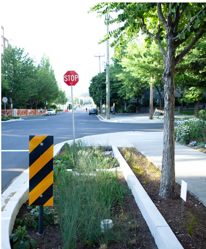
Existing street tree next to bioretention bulge
