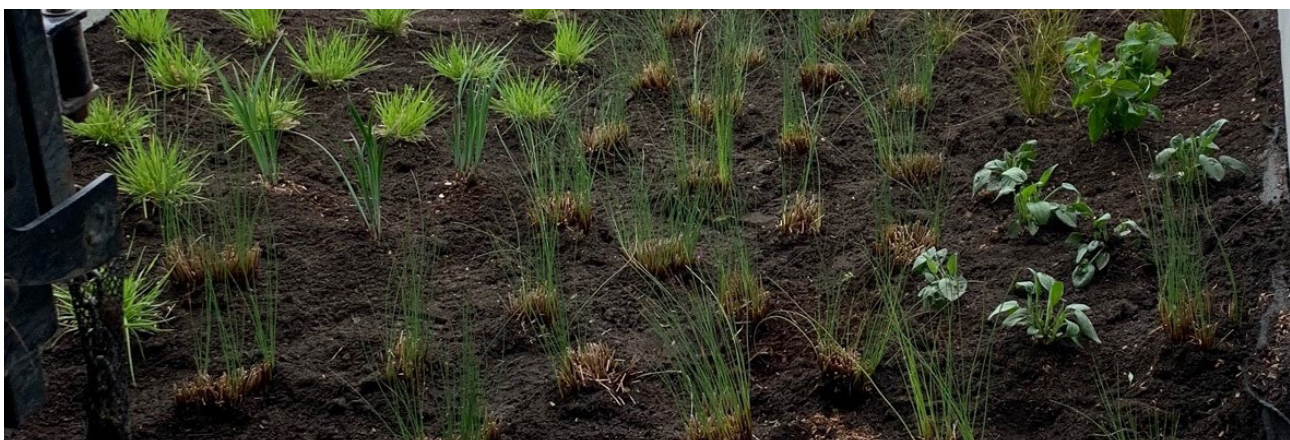
New Planting in Bioretention Soil
