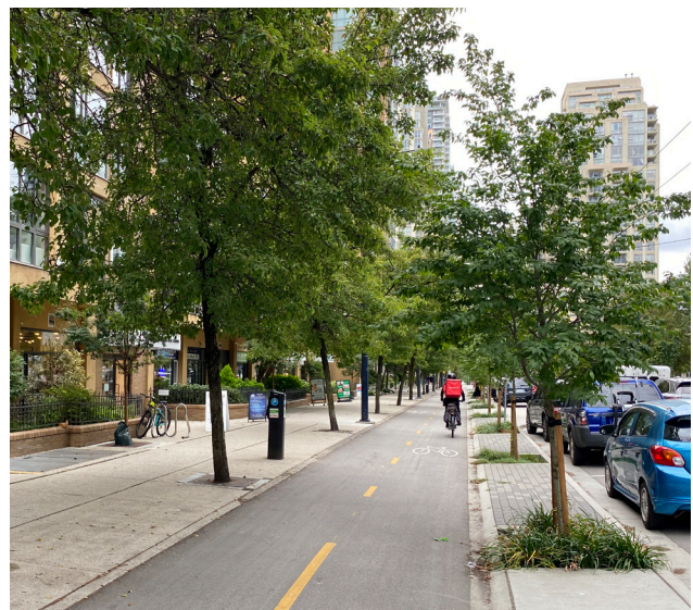
Richards Street Rainwater Tree Trench
