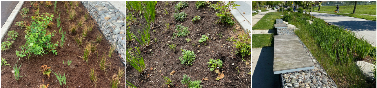
Sunset Park bioswale after planting, at plant replacement 1 year into the establishment period, and the site once fully established.
