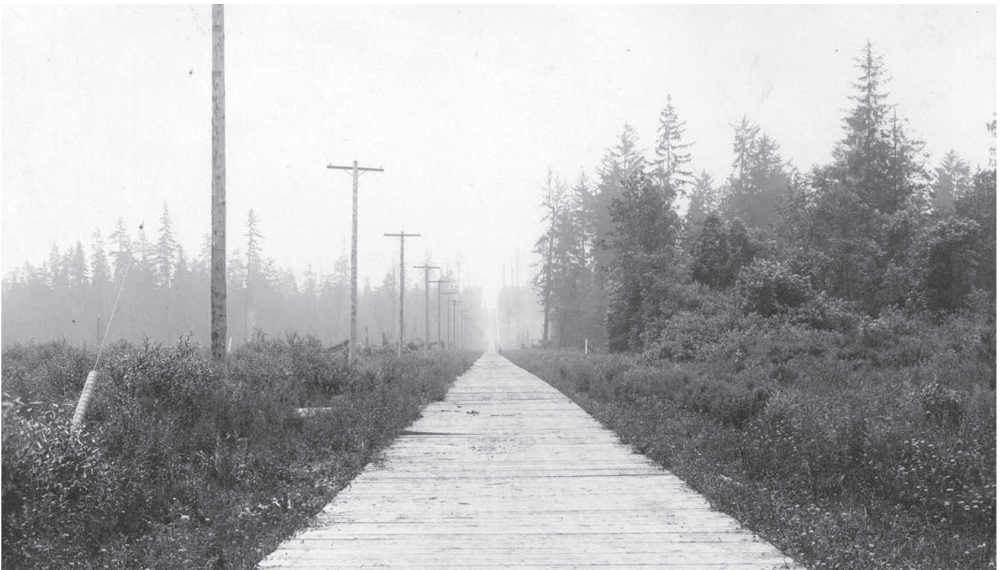
Kaye Road (now Trafalgar Street) plankings by Marshall Plummer & Company Contractors, 1912, City of Vancouver Archives (CVA) Str P207
