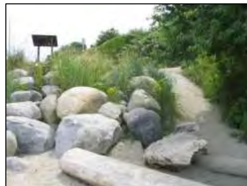
After Construction Showing Successful Foreshore Vegetation Development
