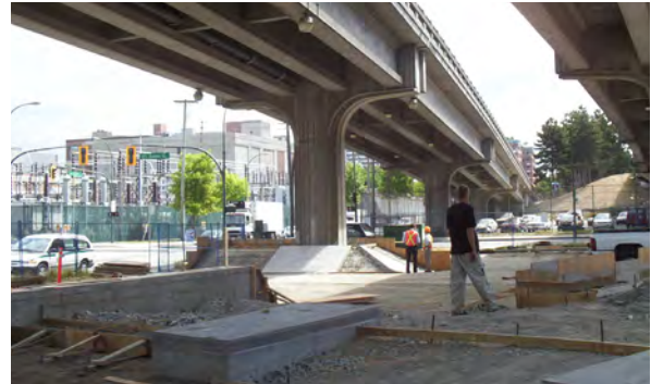
Figure 24. Downtown plaza under construction in 2005
