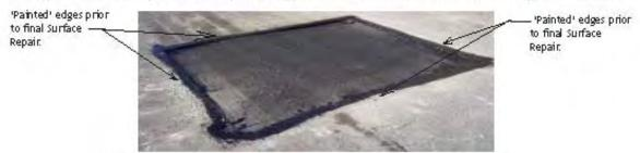
Ensure a seamless joint by 'raking' asphalt fines across the joint & tacked area to fill any voids,
