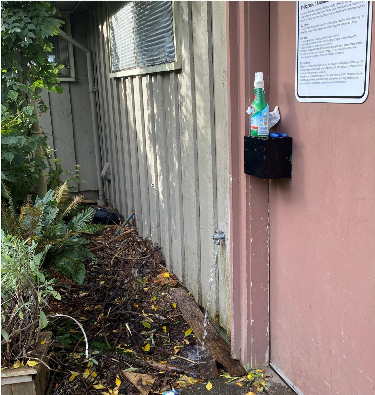
Figure 4. Sampling Station #59 was temporarily removed during construction of the new St. Paul's hospital. Station #59 samples were being collected from a nearby Vancouver Park Board fieldhouse exterior faucet (pictured above) in the interim. This faucet was vandalized, possibly resulting in the total coliform count found in lab samples on October 2, 3 and 4. An investigation in the surrounding area showed presence of total coliforms was restricted to this faucet. Water quality was restored by disinfecting the faucet and flushing.
