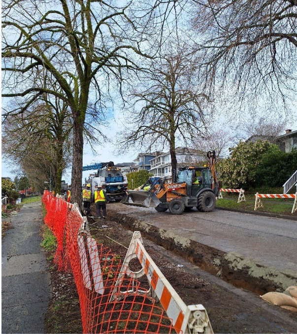
Hastings Sunrise South: Water main construction along East 8 th Avenue.
