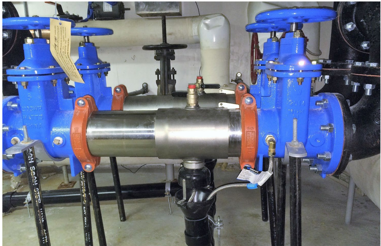
Backflow assemblies are vital components in preserving the integrity and safety of the water supply system by preventing the reverse flow of water and potential contamination.
