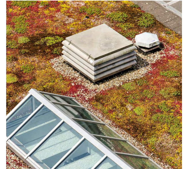
Image (above) - Fire-resistant plant species, such as sedums, are well suited to fire-smart rooftop landscapes due to their ability to thrive with minimal irrigation while retaining moisture within their foliage, helping reduce ignition risk and support resilient planting design.
