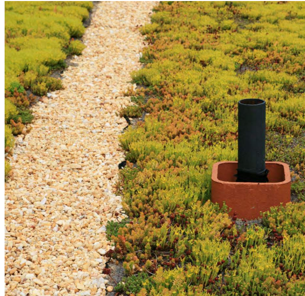
Image (above) - Example of a fire break created using granular materials to interrupt continuous vegetative cover on a roof, helping to reduce fire spread and improve overall rooftop fire resilience.
