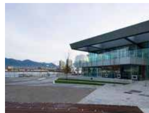
Creekside Community Centre
