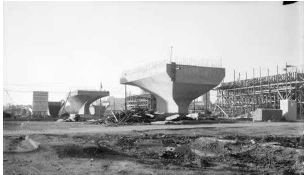
Georgia Viaduct Construction
