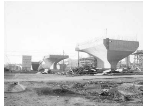
Georgia Viaduct Construction
