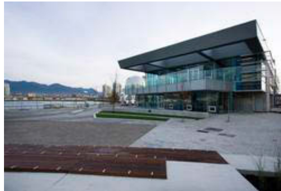
Creekside Community Centre
