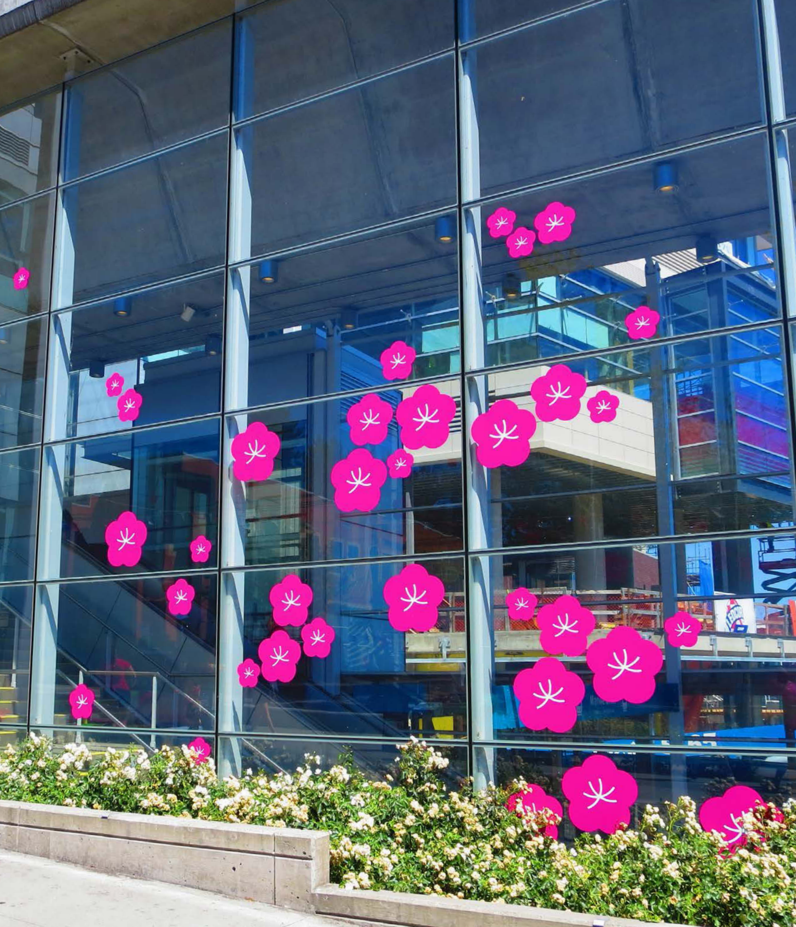
Marine Drive Canada Line Station
