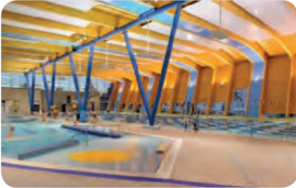
Hillcrest Community Centre | Park Board
