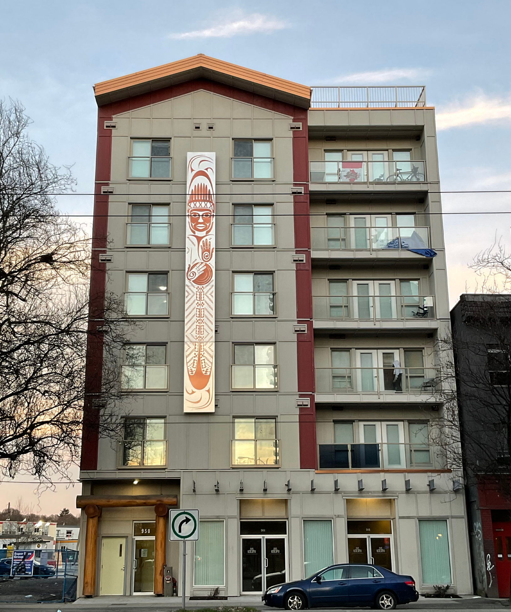
Lu'ma Native Housing Society Social Housing Building
