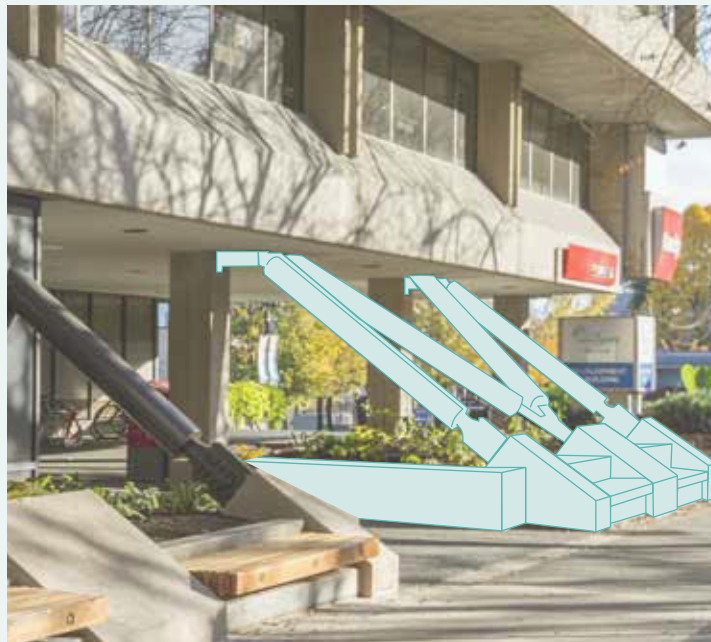
To seismically retrofit the West Annex, engineers use buckling-restrained braces.
