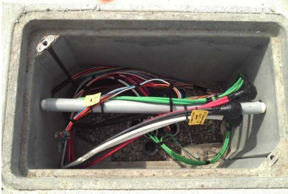
Figure 10-9: Street Lighting Junction Box Example
