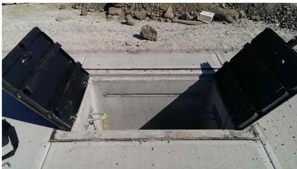
Figure 10-17: Communications Vault
