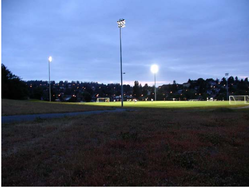
Figure 7– Typical Class IV Soccer Field with LSG Fixtures
