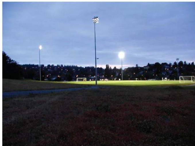
Spill Light Example Urban soccer field with spill and glare control fixtures illuminated to 370 lux with 24m high poles. Photo taken approximately 50m from the edge of the field.
