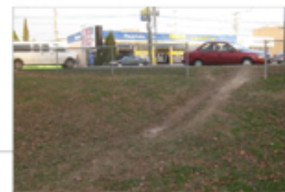
WORN ENTRY PATHWAY
