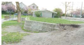
Upper wall raised one block and capped
