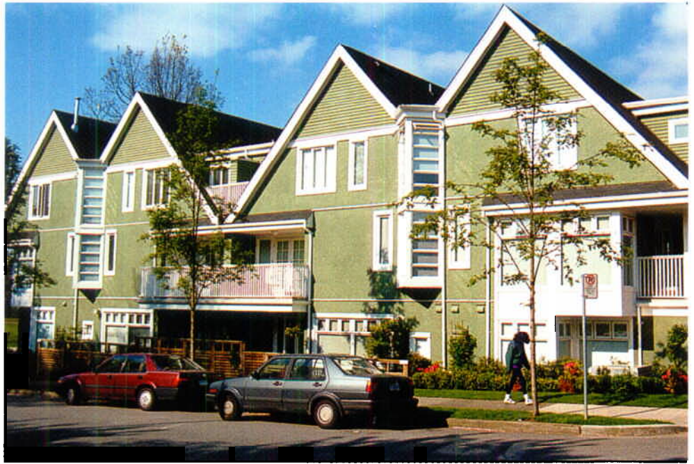
Vine Street 10 unit building
