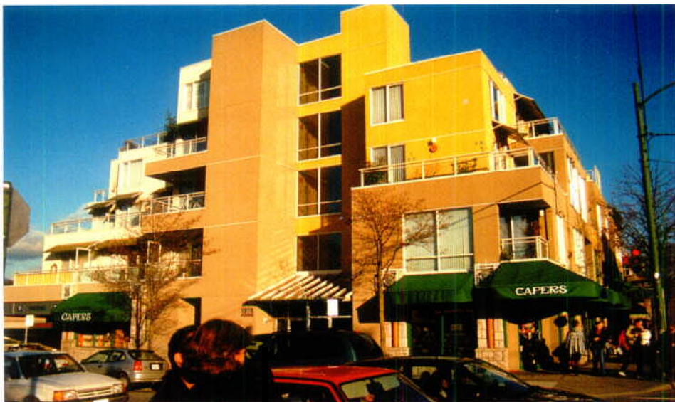
Vine Street terraced massing steps down to respect lower density housing to the north.
