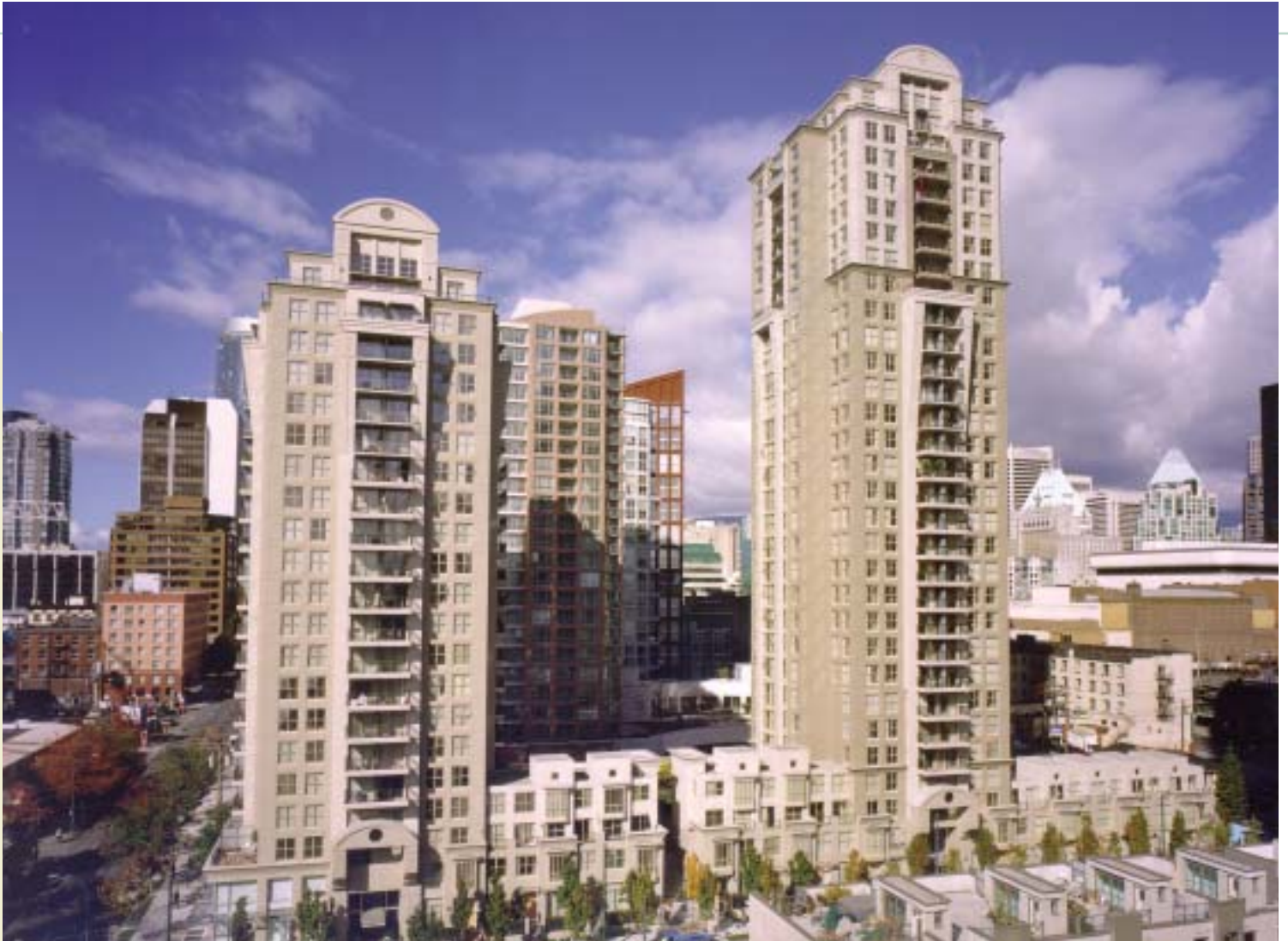
“Mondrian’s” two generously spaced towers integrate with a strong townhouse base along Richards Street and the Contemporary Art Gallery at the Nelson Street corner.
