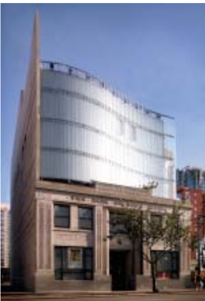
"Scotiabank Dance Centre" incorporates heritage bank facade into contemporary design
