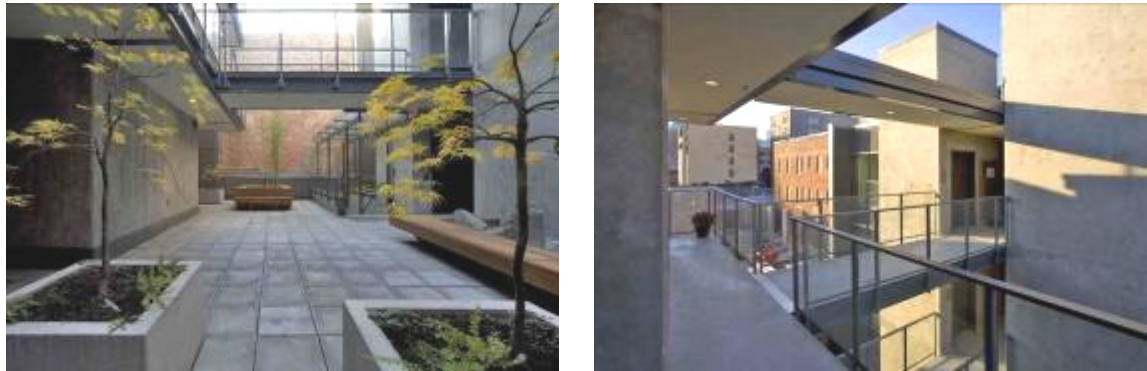
Figure 6. Example of good courtyard with landscaping and careful walkway placement to ensure privacy
