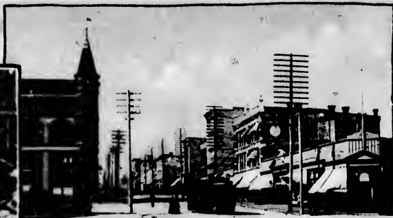
HASTING STREET LOOKING WEST.
