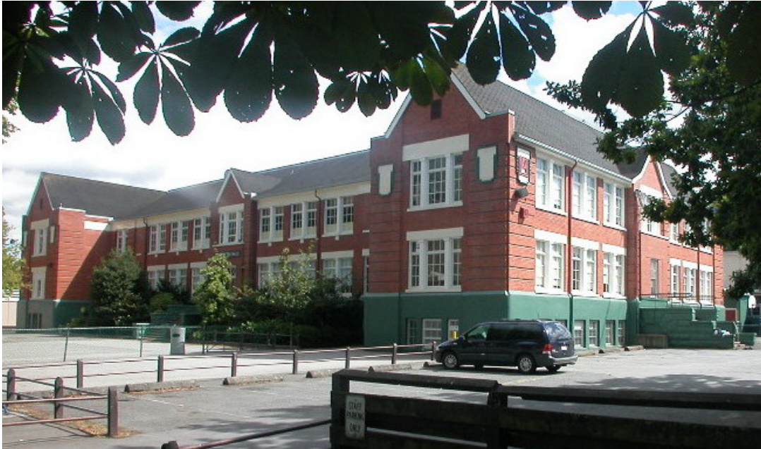
L'École Bilingue, formerly Cecil Rhodes School (1910-12), is an example of a school with restrained classical features and a 'barbell' plan designed by VSB architect Norman A. Leech. (Photo: Commonwealth)
