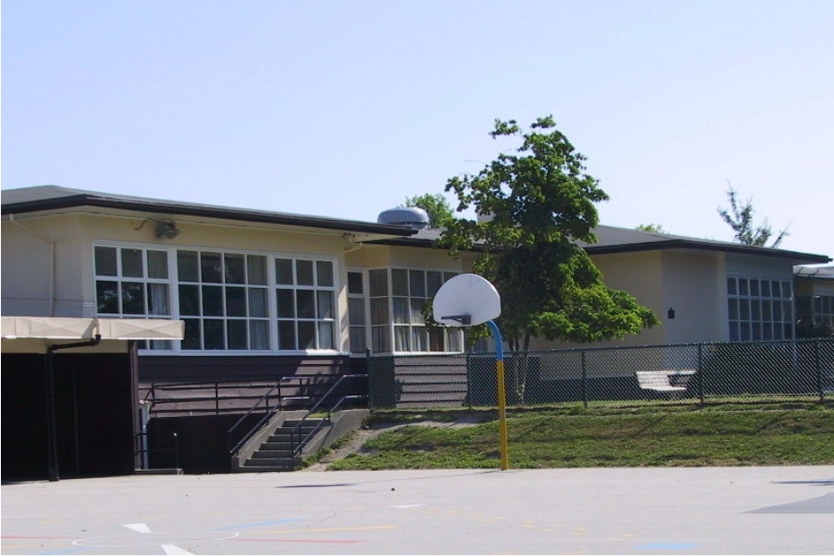
Begbie Annex, now Thunderbird Elementary School, was built in 1945-46 to designs by VSB Architect E.D. King. It was praised as the first school to reflect contemporary ideas about architecture and education. (Photo: Vancouver School Board.)
