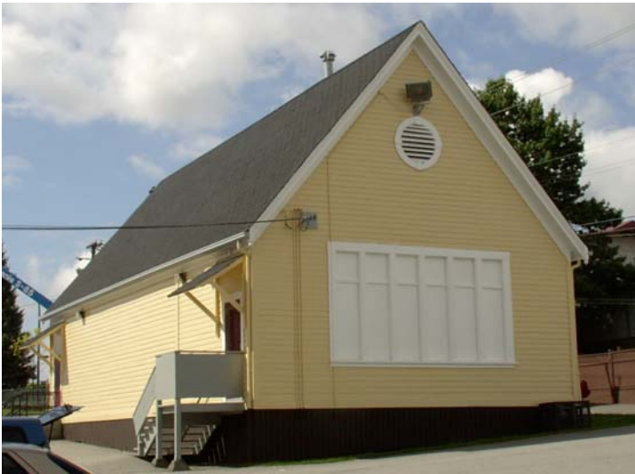
The one-room wood school built in 1896, a component of Sir Guy Carleton Elementary School. (Photo: Vancouver School Board)
