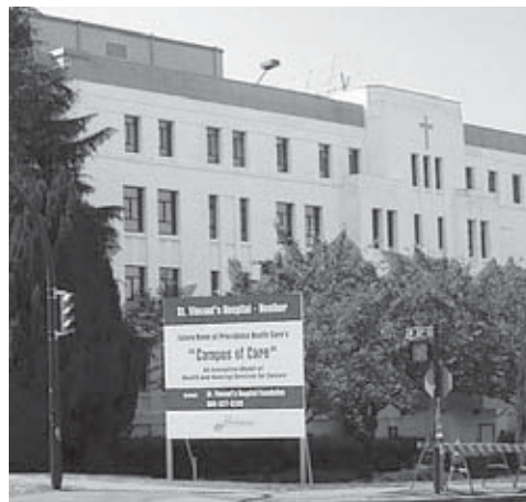
St. Vincent's Hospital Site
