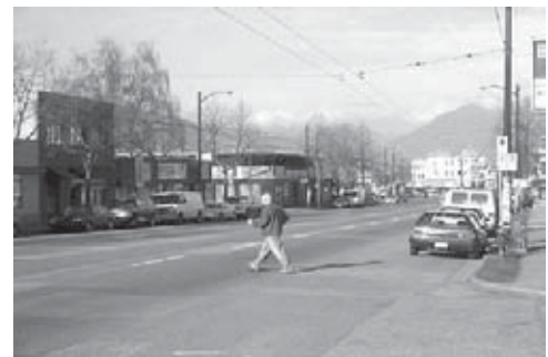
Main Street: Primary arterial needs more and safer pedestrian crossings
