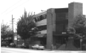
East side of Commercial: office building: no stores at ground level
