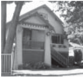
Older character house
