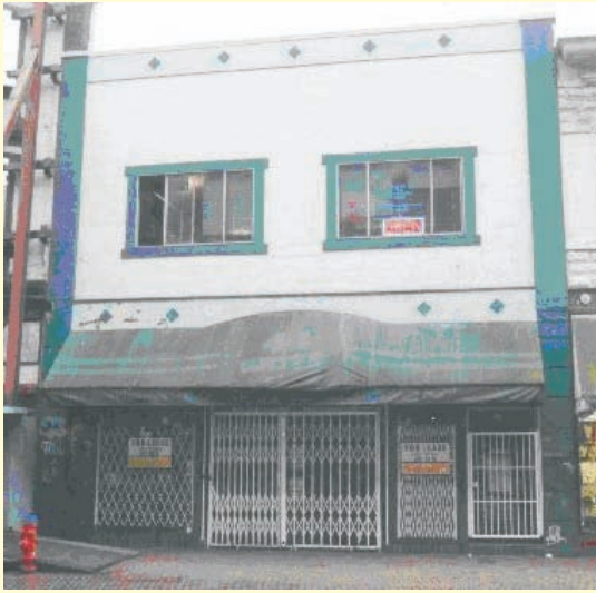
c. 2000 - Before rehabilitation
