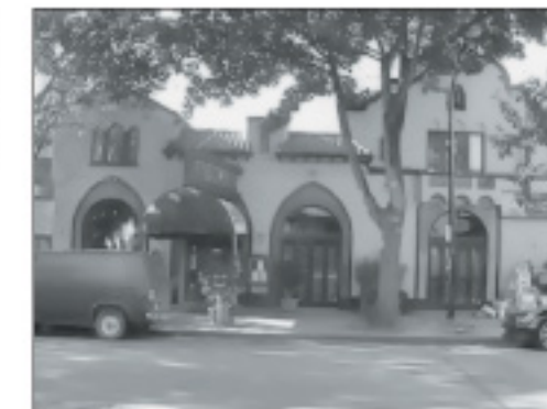
Bidwell street elevation showing McArravy section in centre and left and Lort addition to right
