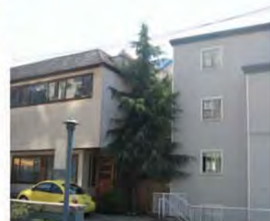
Close proximity and height of building create an unwelcoming entry
