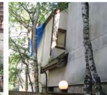
Unattractive dirty two-storey stucco facade will be replaced with a one-storey concrete green wall
