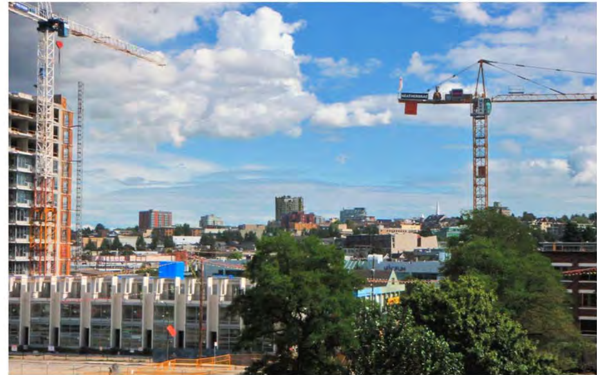
16 view from south end of Cambie bridge
