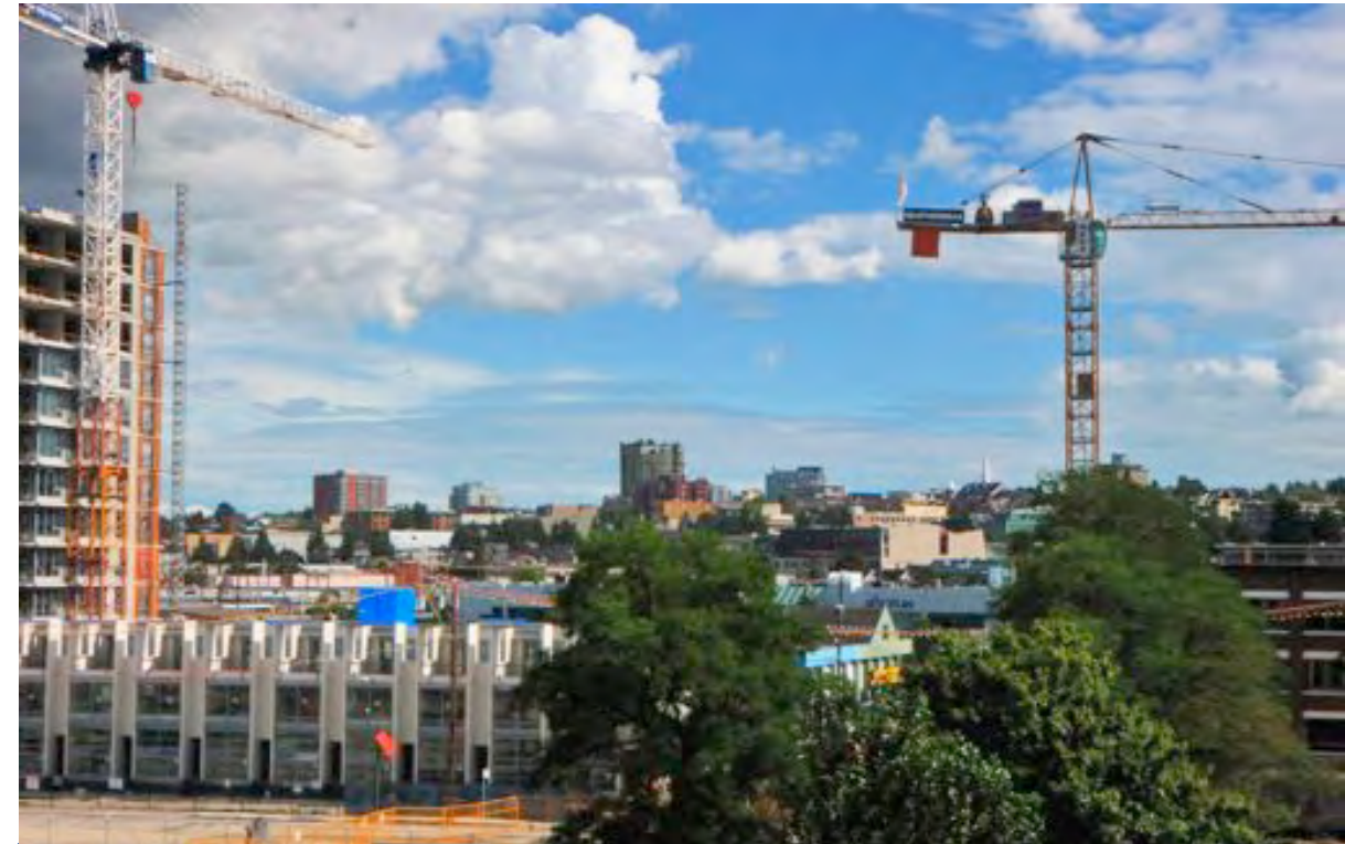
16 view from south end of Cambie bridge
