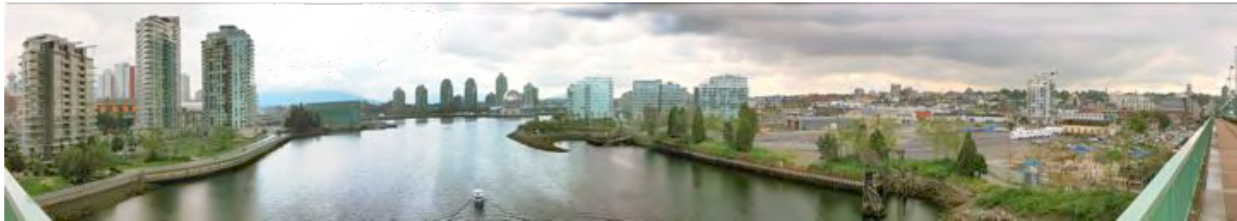
15 view from mid-span of Cambie bridge
