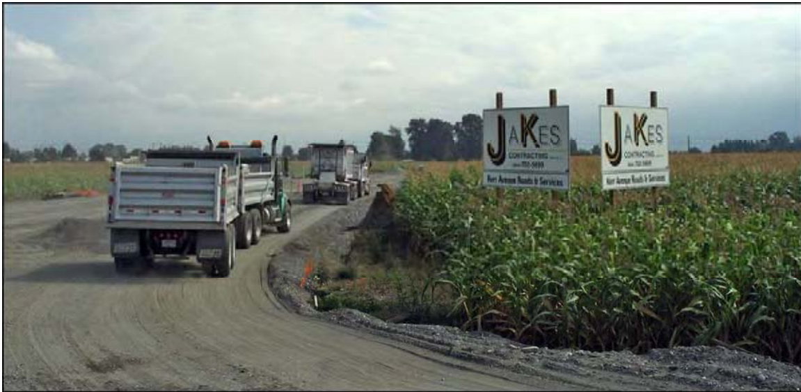
New road on Chilliwack ALR land.
