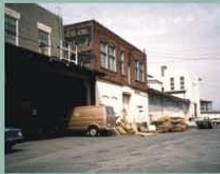
3 - 242 Terminal Ave. Heritage Building Class 'B' Built in 1937
