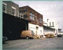
4 - 250 Terminal Ave. Heritage Building Class 'B' Built in 1924
